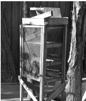
Historic Wilsonia water-cooled "evaporative refrigerator." Originally covered with burlap.
